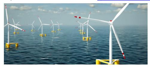
The scope of work covers the FEED for the 190 floating foundations and moorings for the wind turbines and the conceptual design for the floating offshore sub-stations.
