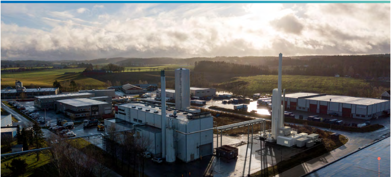
EPF (Engineering, Procurement, and Fabrication) contract by Carbon Centric for a carbon capture unit project in Rakkestad, Norway
