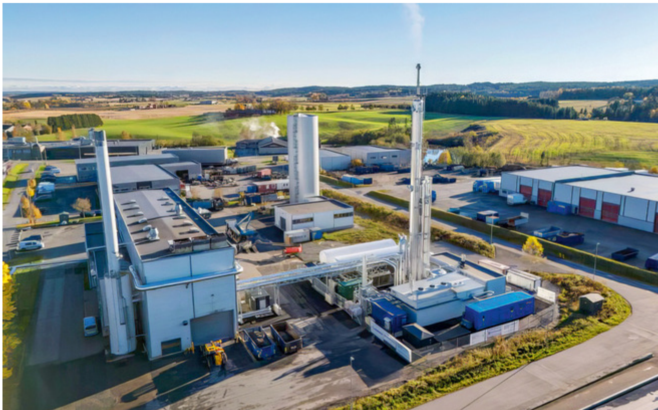
In Norway, the Carbon Centric Rakkestad carbon capture unit, using Technip Energies' Canopy C10 solution, was inaugurated in October 2025.
