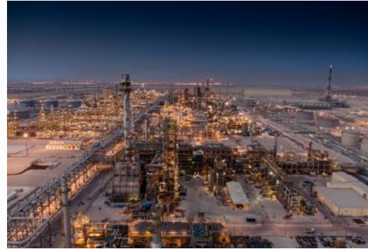
ONE OF THE WORLD'S LARGEST REFINERIES
