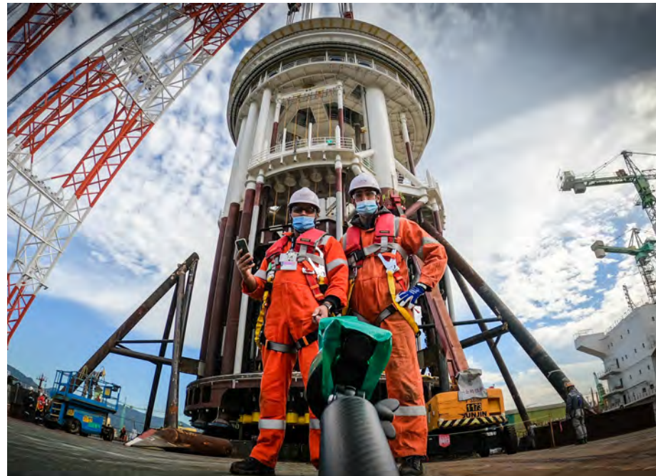
Cybernetix team on Coral FLNG construction yard
